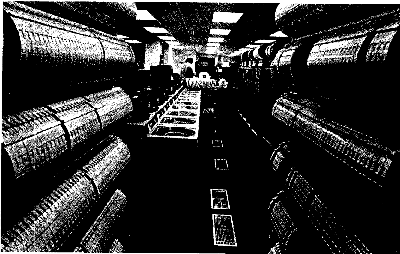
Regulatory data is stored on tape reels and on-line disk files in NASD Data Center in Washington.
